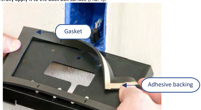
FIG. 4 APPLYING THE OPTIONAL FOAM GASKET TO THE BACK BOX.
