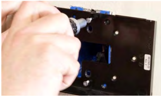
FIG. 5 INSTALLING THE BACK BOX TO THE GANG BOX.
